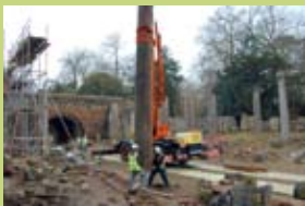
The Ruin during repair
