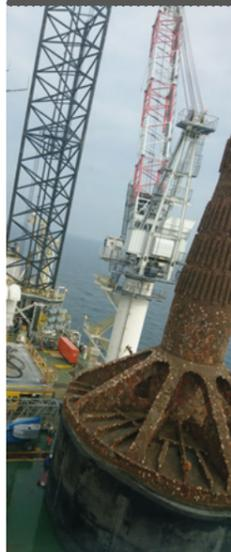
In May 2017 Forewind commenced planning for the decommissioning of its two meteorological masts, situated in the consented Doggerbank Wind Farm. Each meteorological mast stood at a height of 110m above mean sea level and was founded on a suction bucket structure of 50m in length. The larger of the two structures weighed 768t, meaning that there was potential for clay deposits to have built up on the suction bucket structures. If present, these would have impacted the lifting plan.
